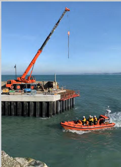
The works were carried out within a Marine Mammal European Protected Species area of concern, as such piling works required specific mitigation measures to be in place. These measures would need to allow impact piling through a body of water in an area containing Harbour Porpoise, Grey Seals along with potentially other protected mammal species sensitive to sound waves.
