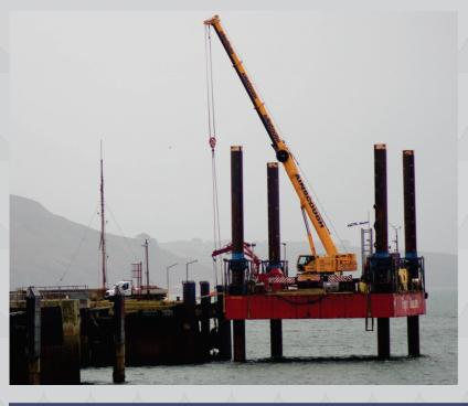
ABP therefore procured a new fender and employed TMS to install it in position. This was completed during March 2017. Due to the loading restrictions on Millbay Pier, TMS mobilised a 250t jack-up barge on which was positioned a 150t crane. The fender was assembled at West Wharf in Millbay before being loaded onto the barge.
