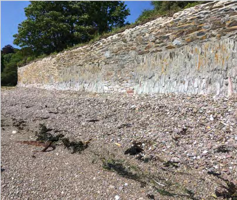
The fourth location, at Mount Edgcumbe Quay itself, was the site of a more serious failure that is currently involving the complete rebuild of an 8m long section of sea wall, using reclaimed limestone and granite blocks. This rebuild is taking the form of a masonry-faced plain concrete gravity retaining wall, much of it being within the intertidal zone.
